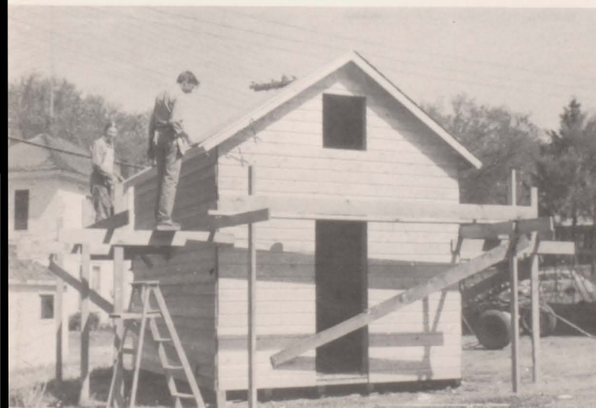
Steve McMullen and Mike Quinn working on a granary in shop.
