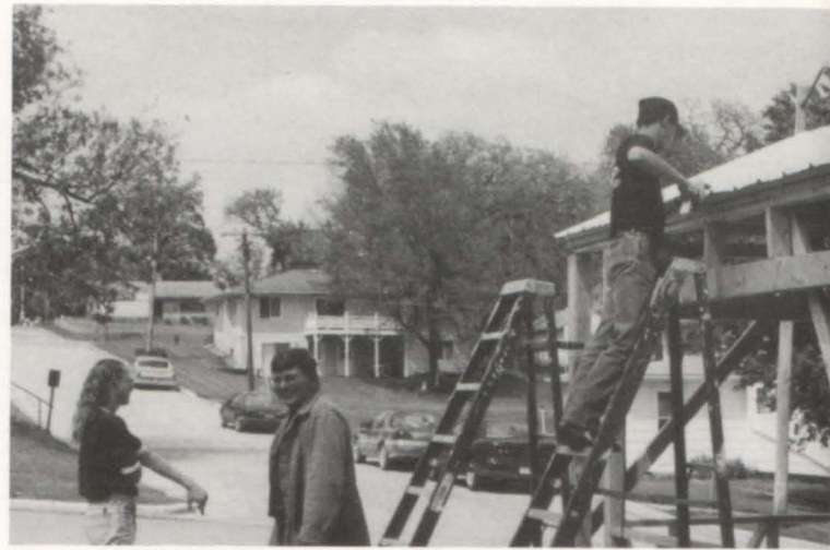
Aaron O'Neill and Mr. Anderson admire the progress of the shed.
